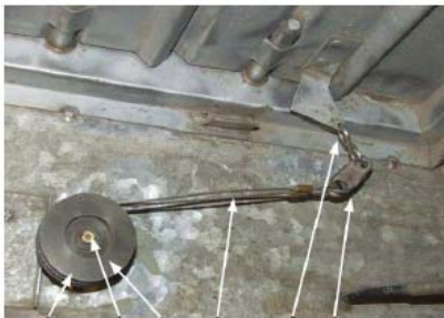
Wrap-spring clutch break Remove and discard old clutch break, shaft, cable, fusible link, and hook.
