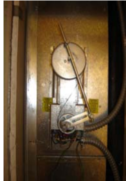
Motor with external springs
