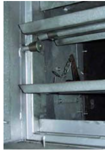
View from inside.
