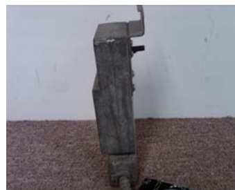
View after removal.
