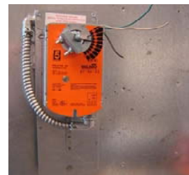
Modern Air Balance has a mounting plate for anti-rotation strap. Some older dampers have actuator hanging in air and a 4x4 box cover plate may be needed for anti-rotation.
