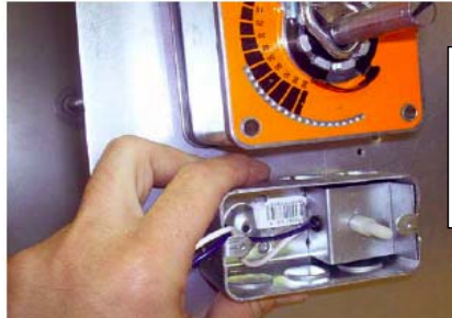
2. Then a new primary thermal sensor must be installed to control the actuator electrically.
